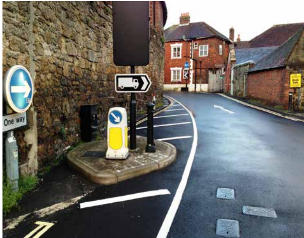
Excessive markings and clutter - Petworth
