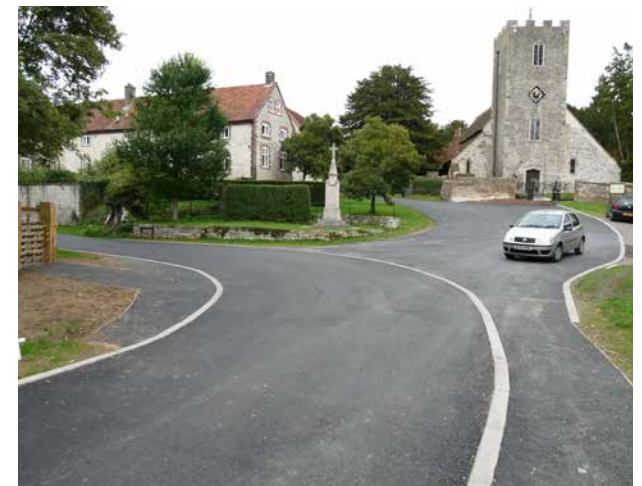
Sensitive highway treatment - Buriton, Hampshire
