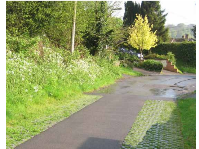
Reinforced grass paving forms soft verge - Buriton
